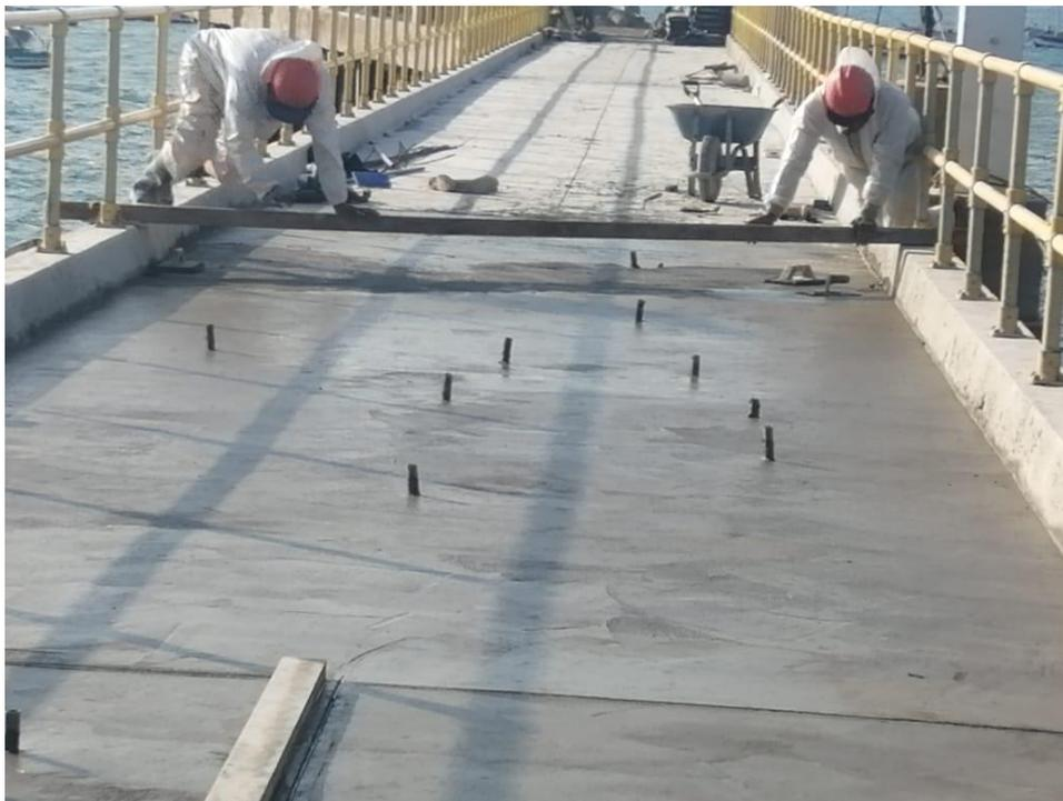
VACEADO DE CONCRETO FIBROREFORZADO F'C=350KG/CM2
