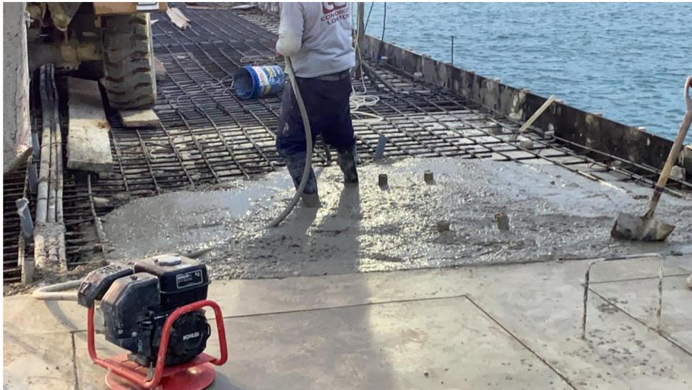
VACEADO DE CONCRETO FIBROREFORZADO F'C=350KG/CM2
