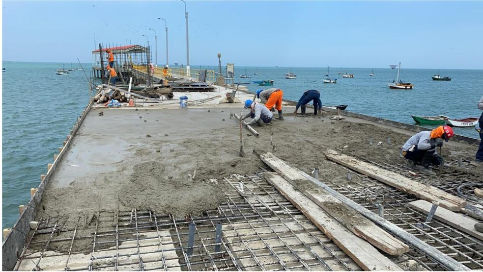
VACEADO DE CONCRETO FIBROREFORZADO F'C=350KG/CM2
